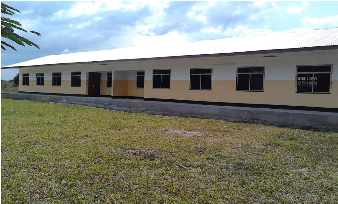
Construction of Laboratory at Mabwepande Secondary school
