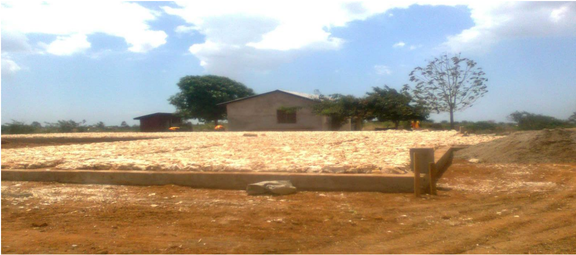
Construction of Administration Block Malolo Agricultural Centre
